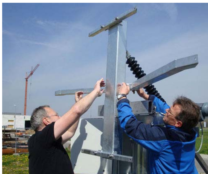
Figure 6-4: Mounting the crossbar
